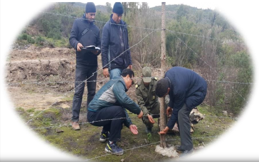
Inspecting of construction status
